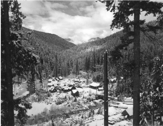
Figure 1. Jawbone Flats, OR in the Opal Creek Wilderness Area in 1947, showing many of the buildings used in this study. Photograph provided by Tom Atiyeh.
